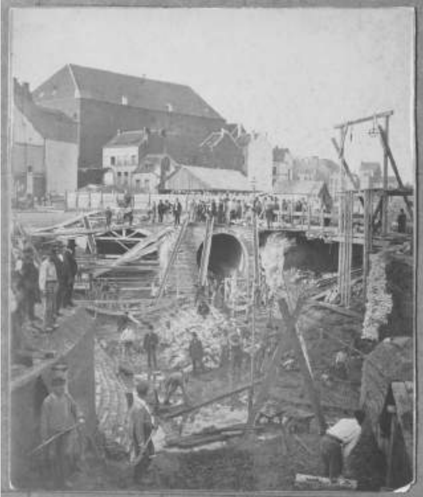
Sewage construction works and vaulting of the river Senne (ca. 1870), BCA (CI F-1441)
