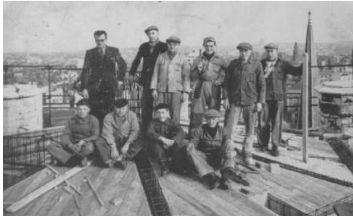
Construction workers on a roof in Brussels, ca. 1940 (BCA, CI-C1165).
