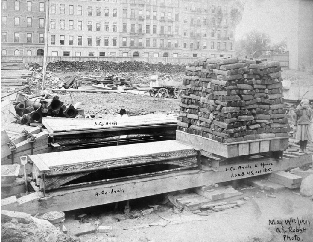
Test of a tile vault (Guastavino Fireproof Construction Company architectural records)
