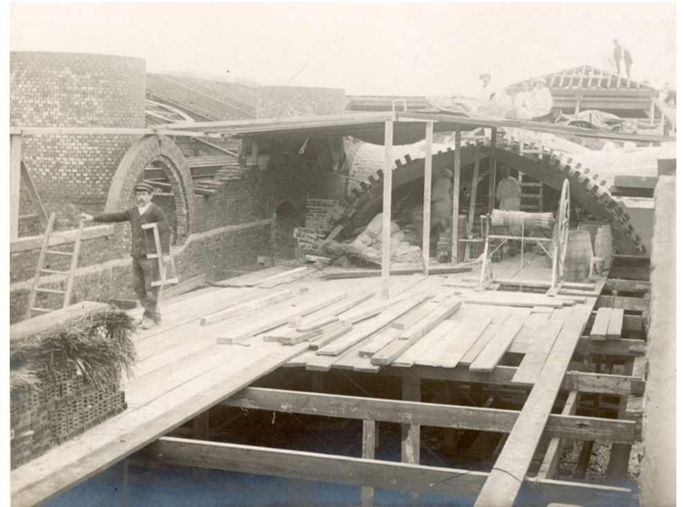
Construction of the vaults of the lateral galleries in the Royal Museum for Central Africa (Source: HP.1968.10.6-43, RMCA Tervuren collection, Charles Girault archives)
